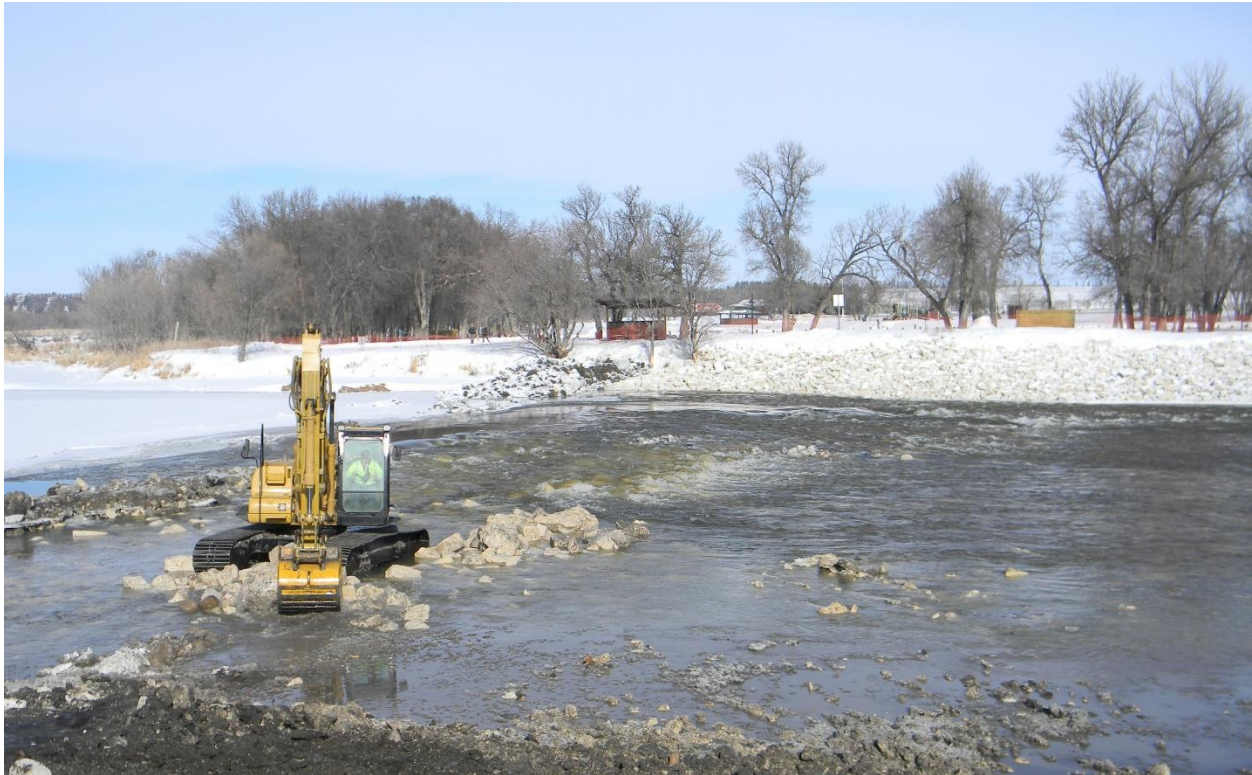
Original Construction Photo 1: Placement of rock dam core
