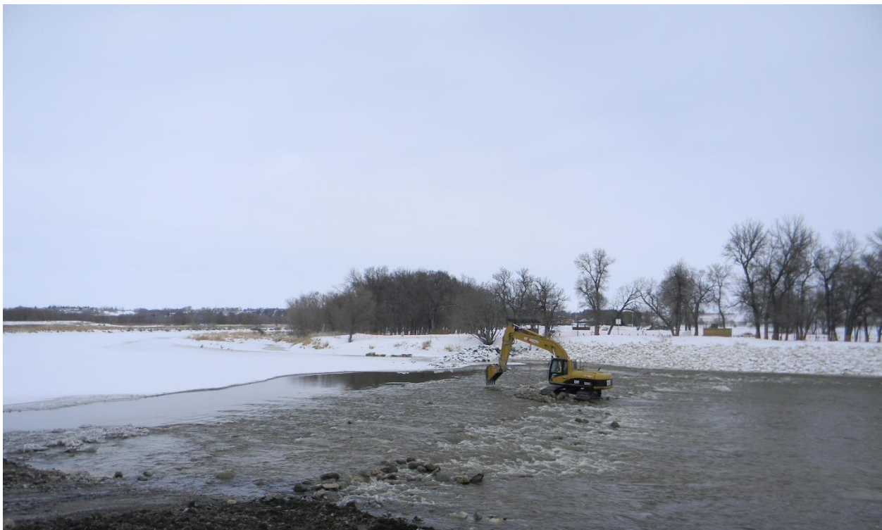
Original Construction Photo 2: Final grading of rockfill
